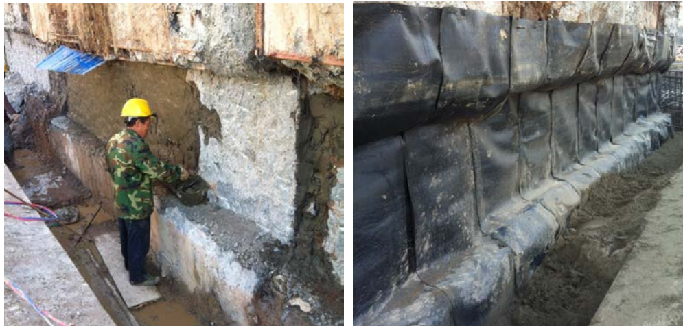
(a) Level the groove
