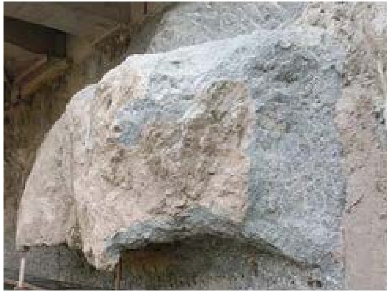
Figure 6: Local failure of slurry trench
