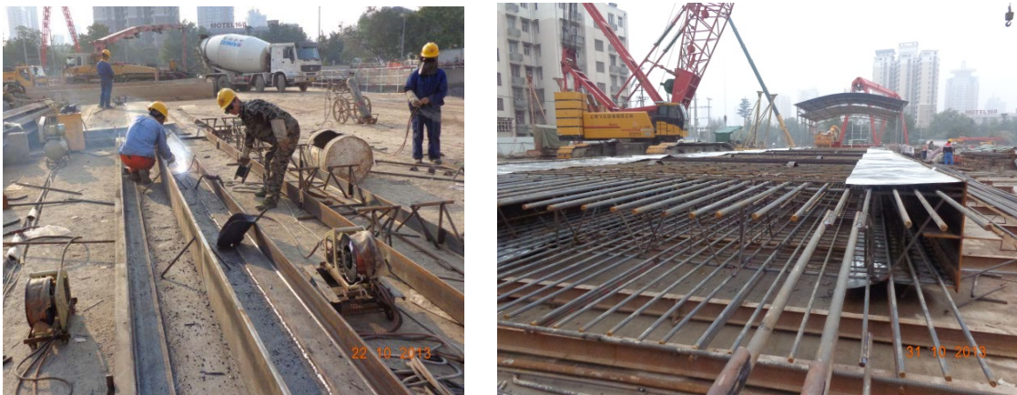
Figure 5: The picture of cross-steel joint
