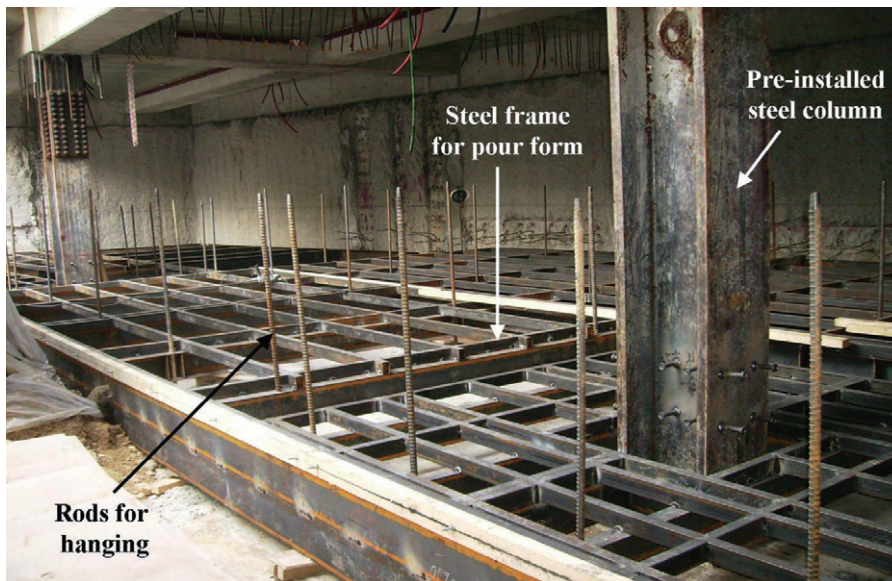
Figure 15. Steel frame supporting pour form with rods
