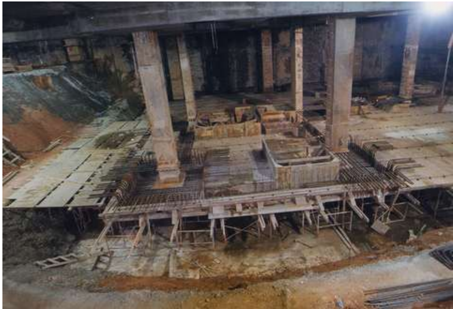
Other work reality in top-down basement – congested work environment, complicated layout, difficult phasing of work as part of the construction planning
