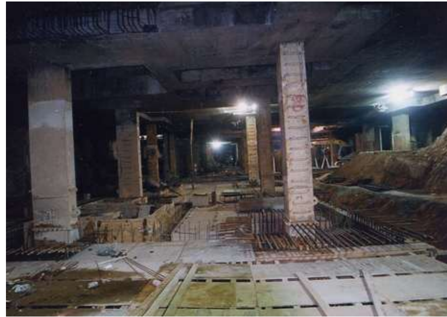
Other work reality in top-down basement – congested work environment, complicated layout, difficult phasing of work as part of the construction planning
